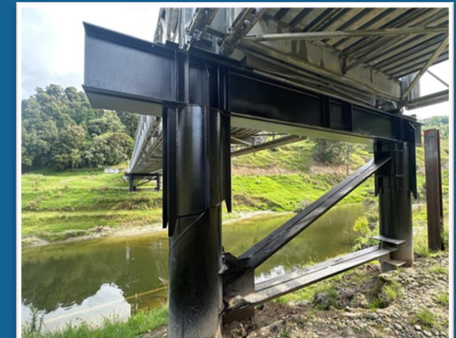
Hollywood strengthening complete.
