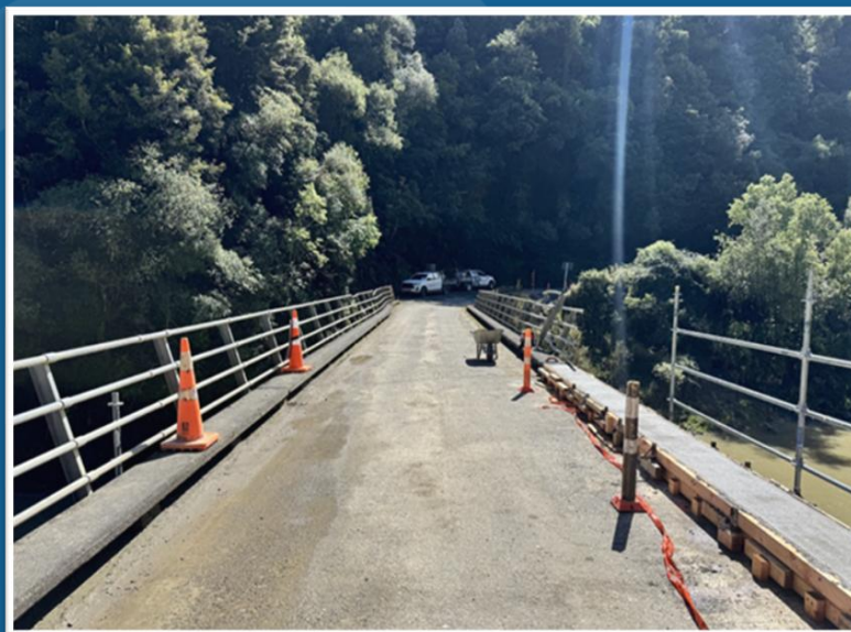
Ruakaka repairs underway.
