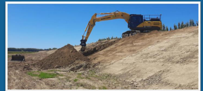
Waipaoa Stopbank construction
