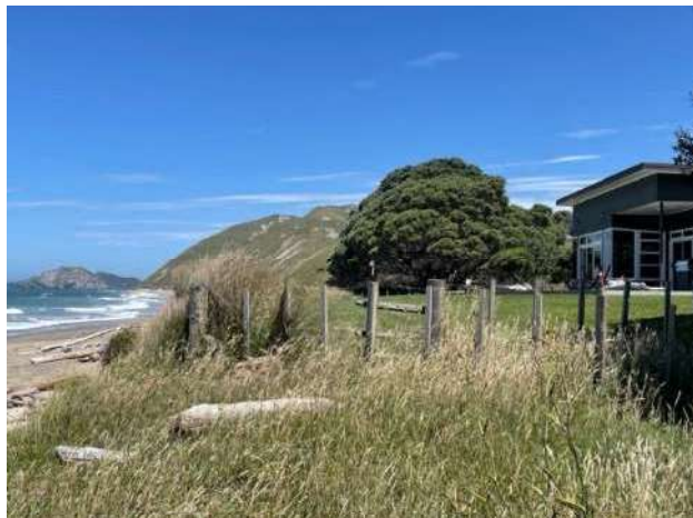
Photo 1: proximity of proposed Trail to property
