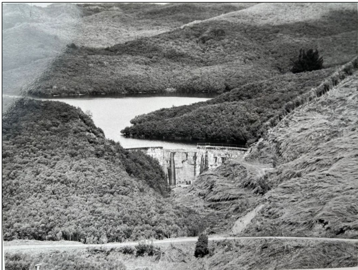
Figure 21: No. 1 Clapcott Dam, 1982. 91
