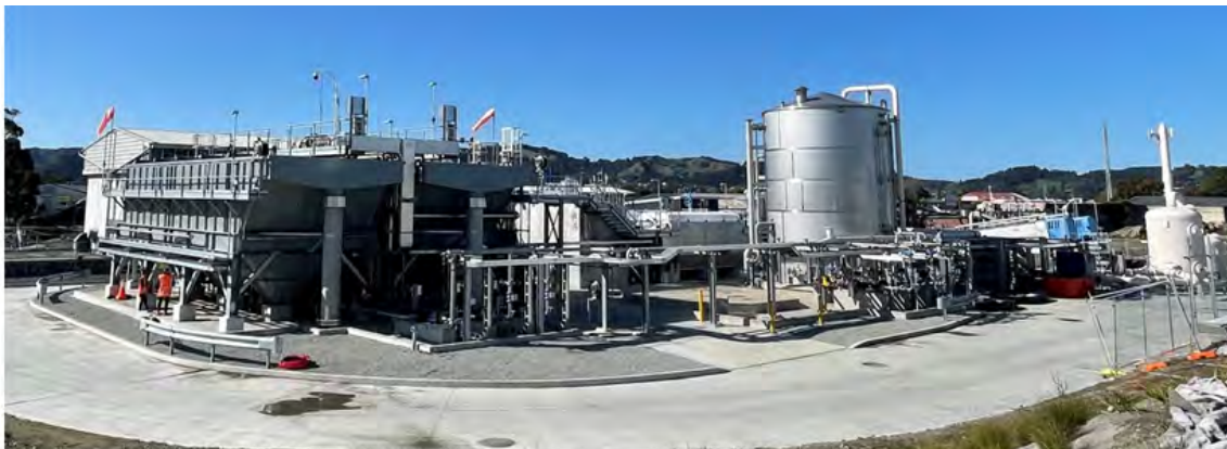
Banks St Wastewater Treatment Plant, Stage 2
