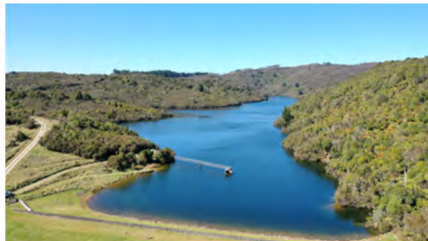
HC Williams Dam, one of the three Mangapoike dams
