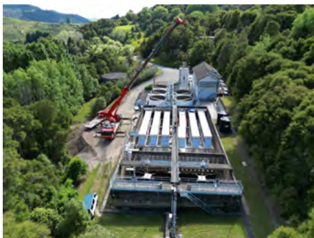
Lamella filters being installed at Waingake Water Treatment Plant
