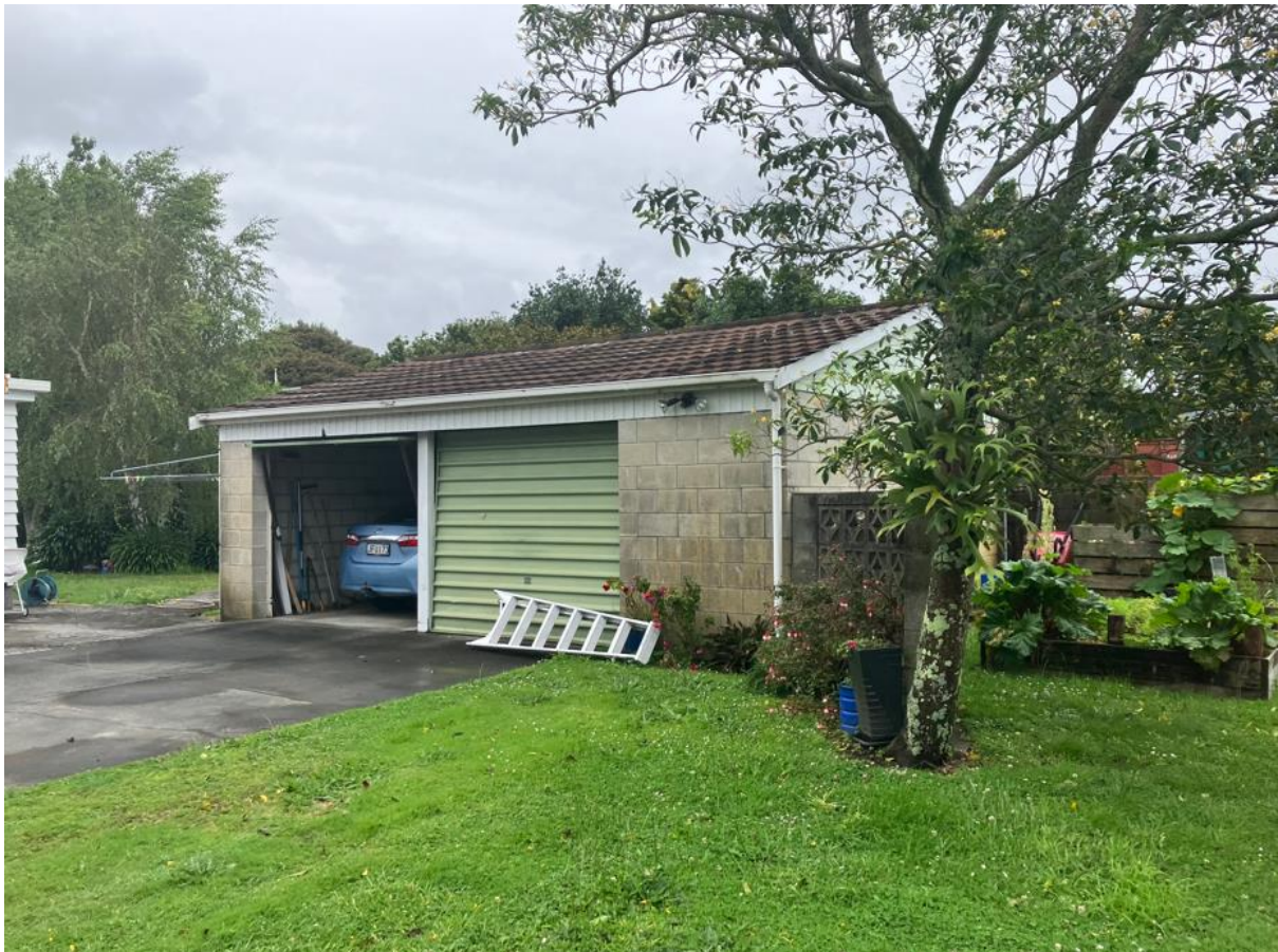
Image 10 – Facing west: The existing garage.
