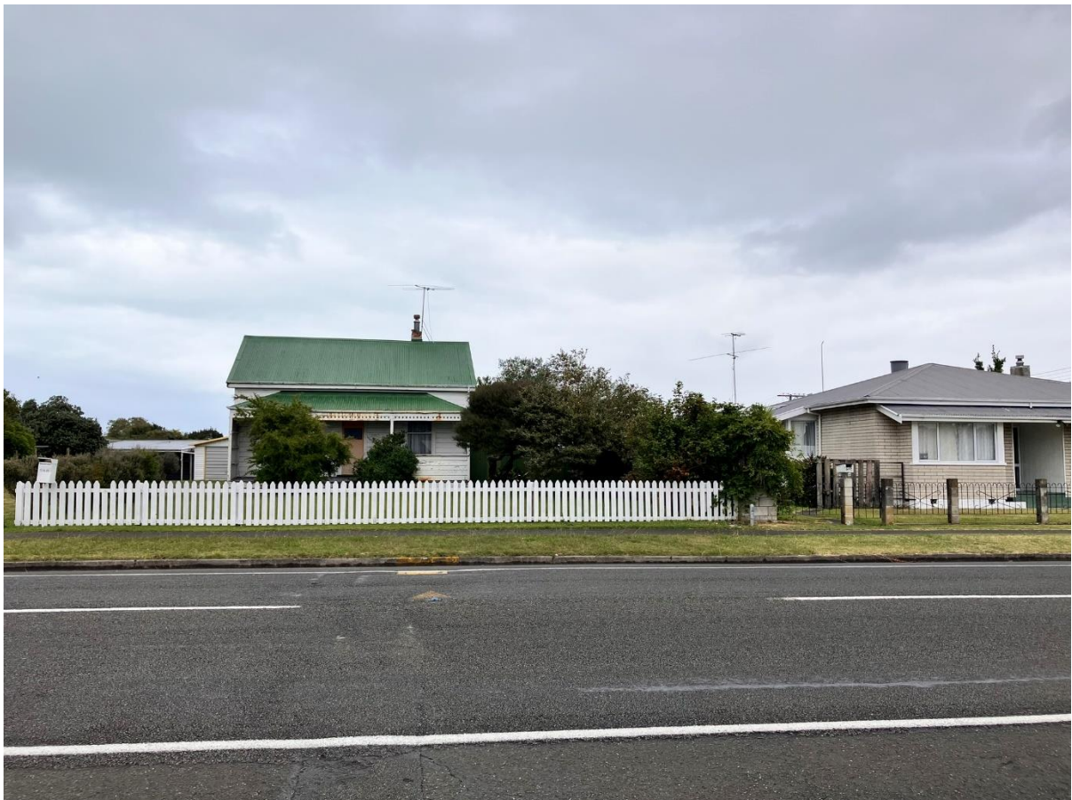
Image 11: Facing south: the subject site at 560 Aberdeen Road.
