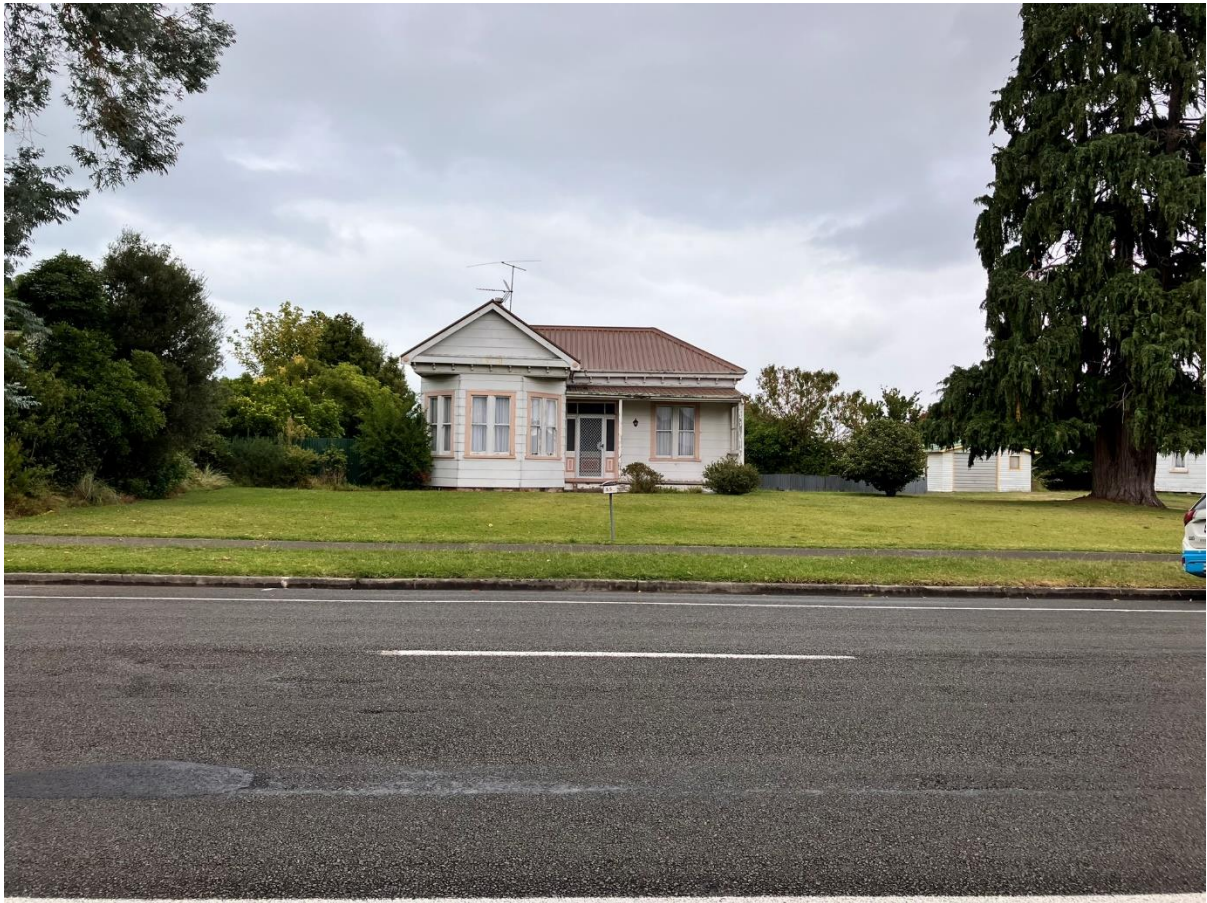
Image 6: Facing south: the subject site at 556 Aberdeen Road.
