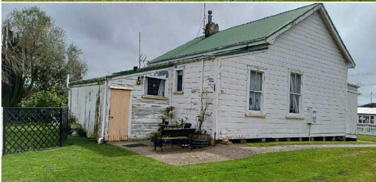
Top. Front of 560 Aberdeen Road. Middle. Sheds on eastern boundary of 560. Bottom. Photo looking north-west at side of dwelling on 560 Aberdeen Road.
