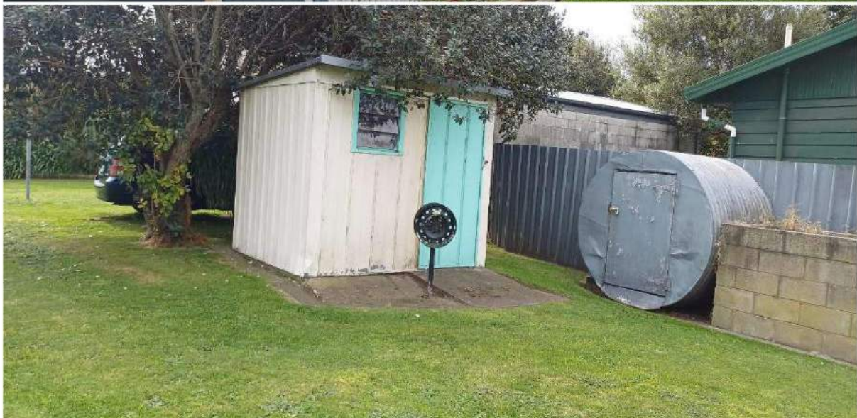
Top and middle. Large garage in far south of 556 Aberdeen Road. Bottom. Small garden shed on 560 Aberdeen Road.
