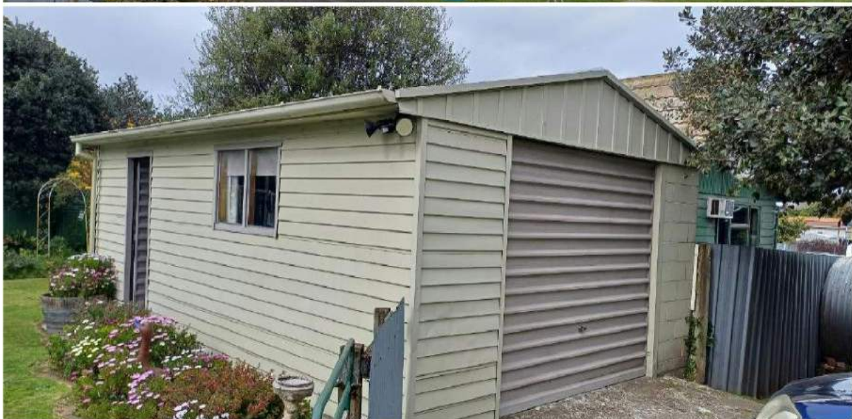
Top. Looking east towards rear of dwelling on 556 Aberdeen Road. Middle. Back of 560 Aberdeen Road dwelling. Bottom. Garage at 556 Aberdeen Road.
