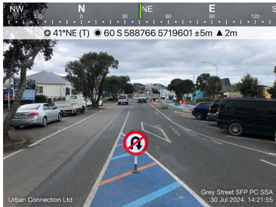
Figure 4.4-31 – Faded centre lines on Grey Street in front of the skate park
