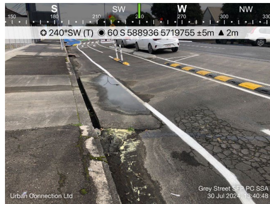
Figure 4.4-41 – No green surfacing through driveway
