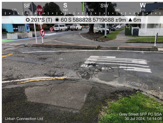
Figure 4.4-36 – Pavement defects
