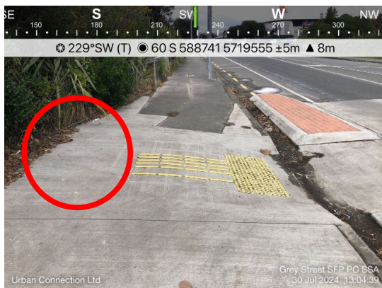
Figure 4.4-15 – Directional tactiles do not cover the entire footpath
