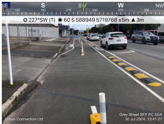
Figure 4.4-40 – No green surfacing through driveway
