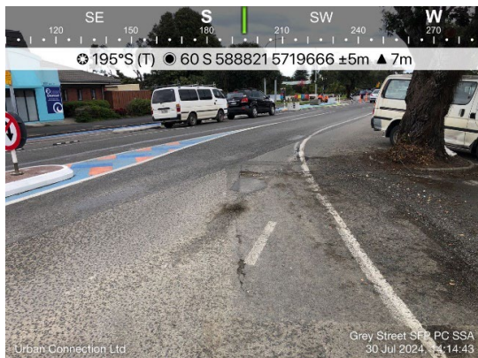
Figure 4.4-38 – Pavement defects
