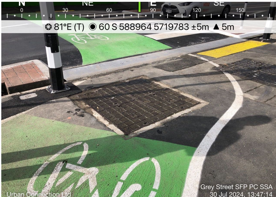
Figure 4.4-28 – Manhole cover on the cycleway
