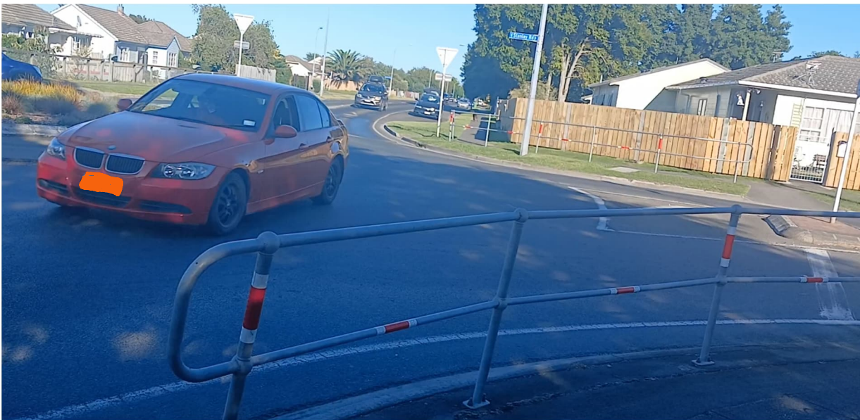
Figure 18 Safety Handrailing at Childers Traffic Circle to protect pedestrians
