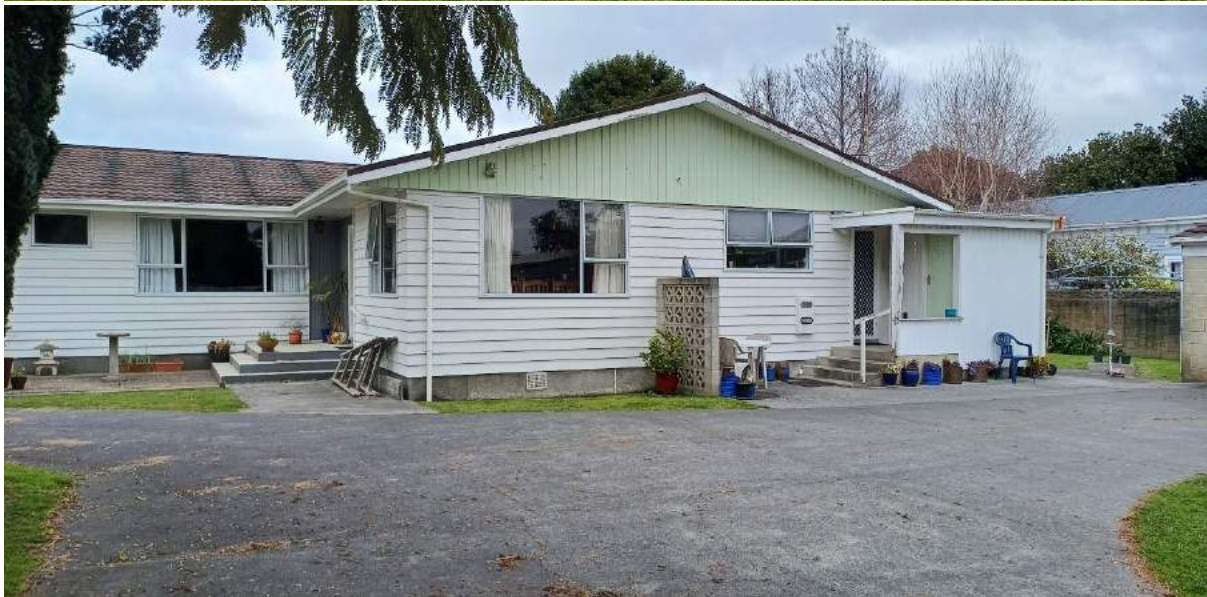
Top. Asbestos construction on porch Middle. Northern side of property. Bottom. North facing side of house.
