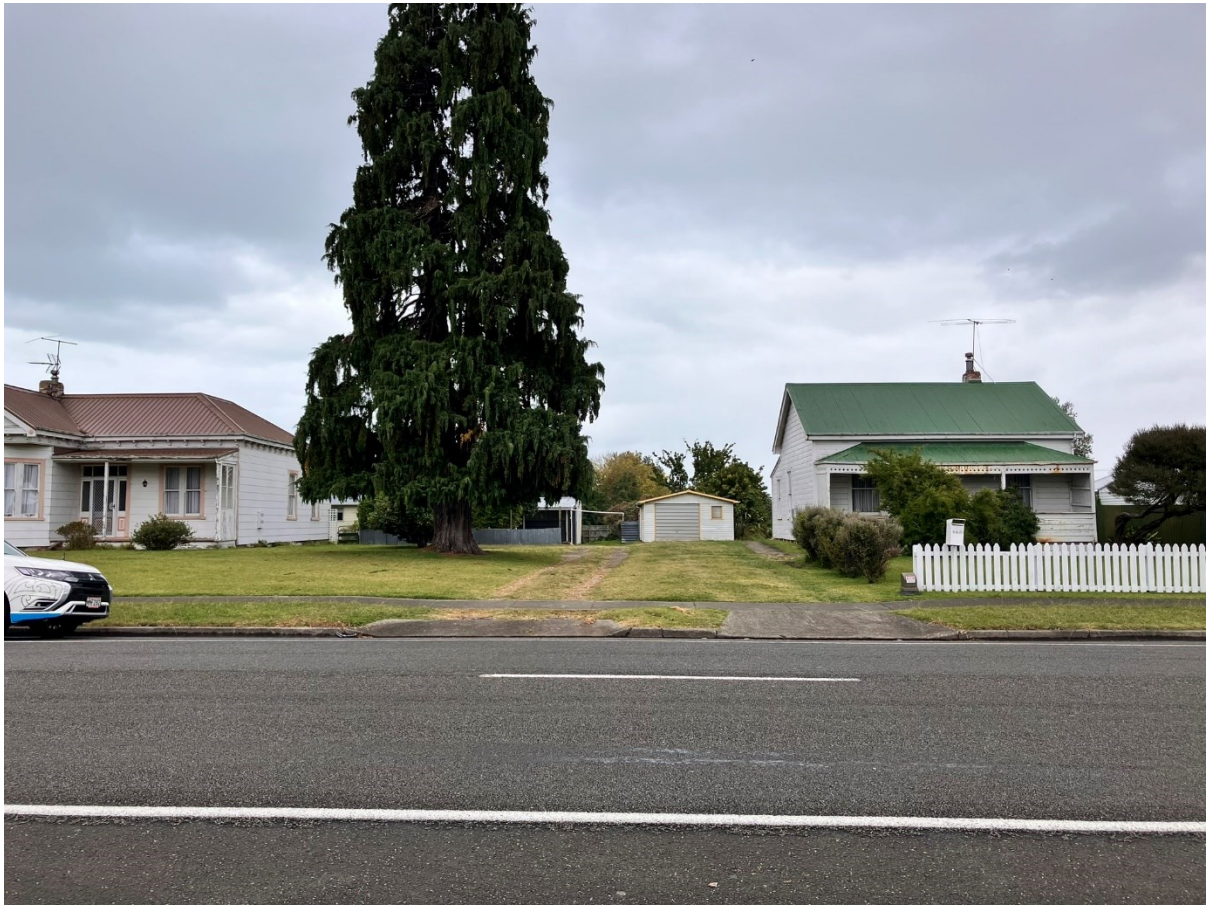
Image 16: Facing south: the subject site at 556 Aberdeen Road to the left and 560 Aberdeen Road to the right.
