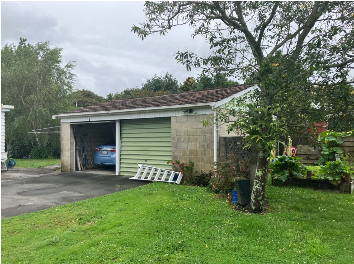
Image 9 – Facing west: The existing garage.
