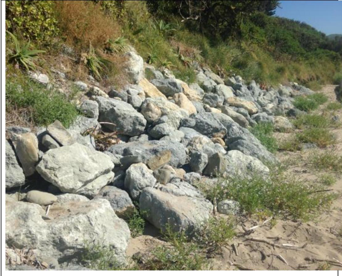
**Figure 1-** Rock revetment on Wainui Beach comprised of locally sourced boulders, which are degrading due to wetting and drying in a supra-littoral environment.
