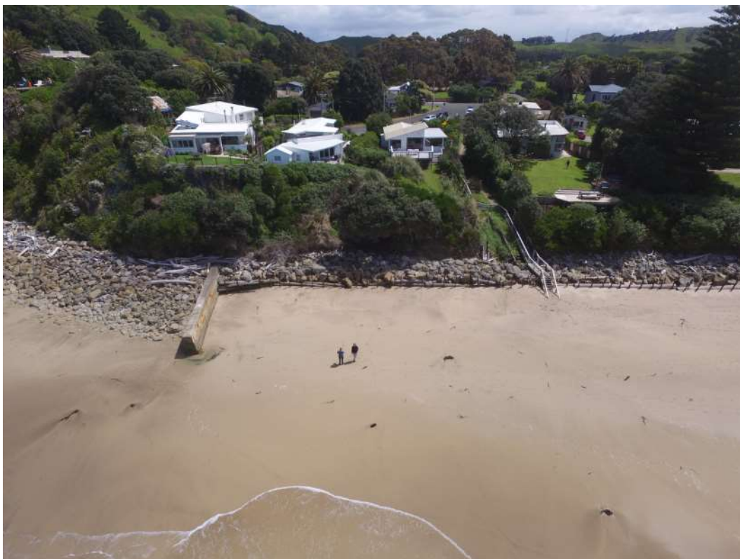
Figure 1 Location of proposed rock revetment between the existing concrete groyne and Tuahine Crescent accessway
