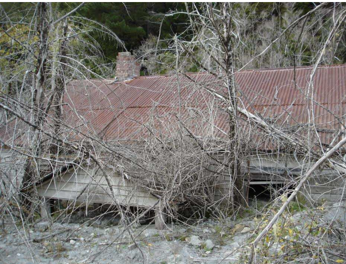
Fig. 11: The whare, partially buried by gravel and silt from Barton's gully. Photo: Courtesy of Dr. M Marden; photo date: 2009.
